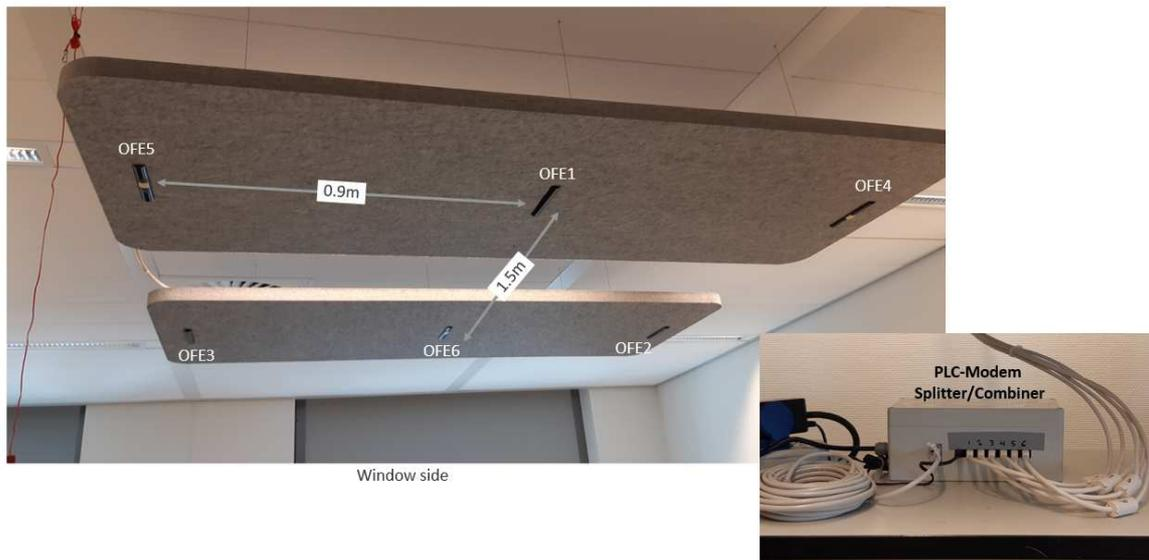
Figure 2: Office demonstrator: ceiling LIFI-MIMO installation
