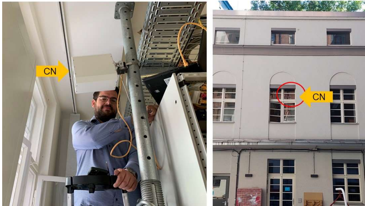
Figure 4 OWC client node (CN) installed inside the building (behind the window).
